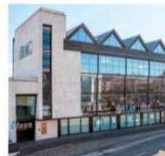
Headquarters: Banca Agricola Commerciale S.p.A.
